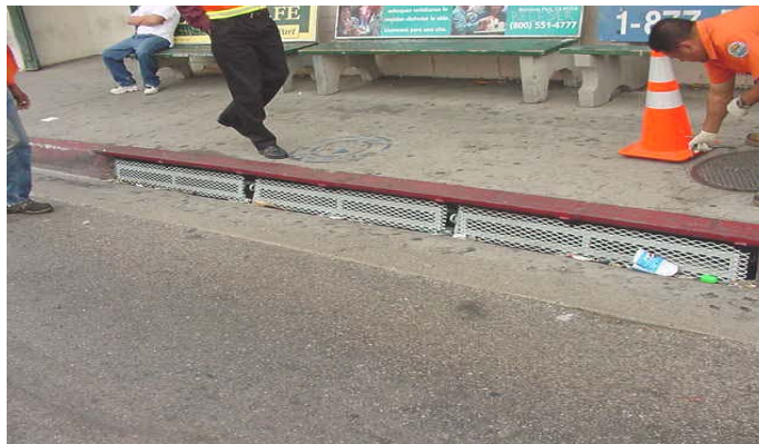
Installation of catch basin insert to prevent debris entering into
