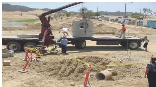
Installation of storm drain insert device to treat storm water
